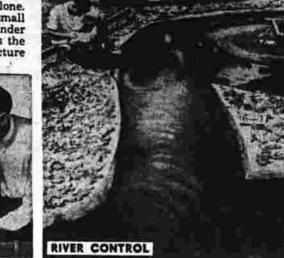
Since rivers often are more temperamental even than machines, engineers use miniature streams to test proposed changes in course. This model paved the way for a cut-off in Mississippi.
